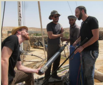
The team installing the SMPP
